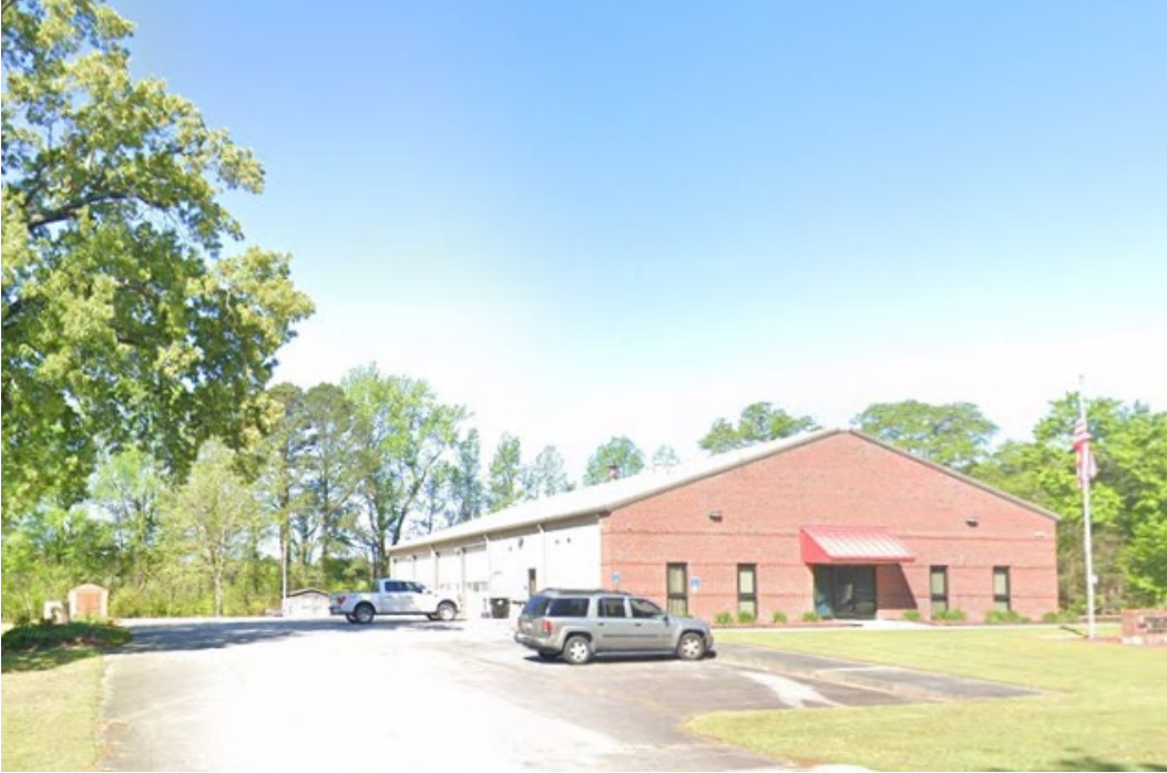
Fountain Rescue and EMS building
